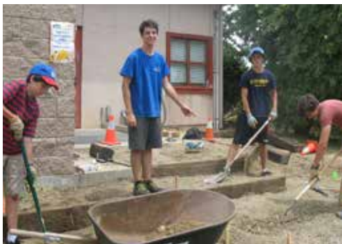
Nick Grabert (in blue) and his fellow Scouts building the new walkway.
